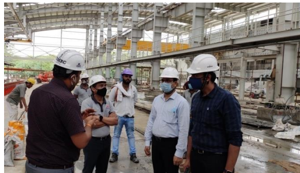
Photo 7: Er. Rishi Gangwar, Chief Engineer (Civil Works) (First from Left) explaining the ongoing work to the envoy with Project Director, Er. Arvind Singh (Second from Left)
